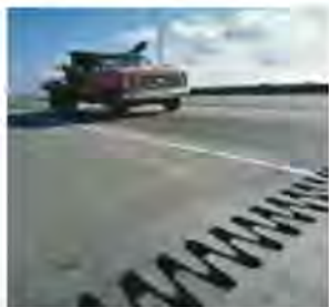
FIGURE 17-3 Expansion joint on a bridge.
