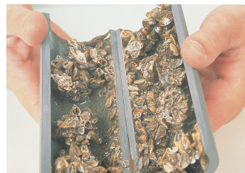
Figure 11-CS11_01 Zebra mussels clog pipes.
