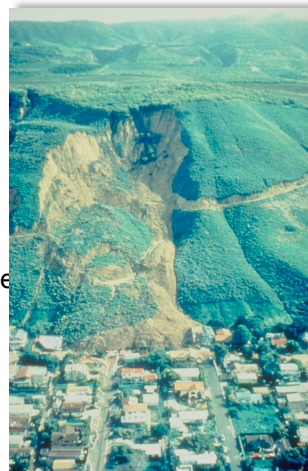
Landslide and Debris Flow, La Conchita, California
